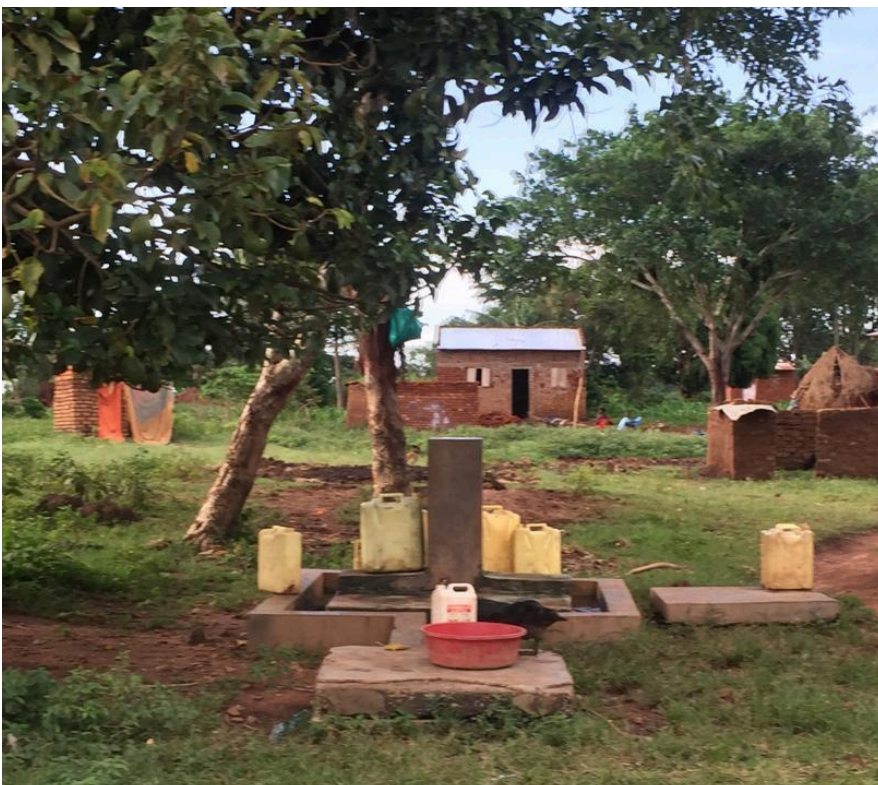
One of 17 solar-fed taps delivering clean water for household use in Namutumba.
