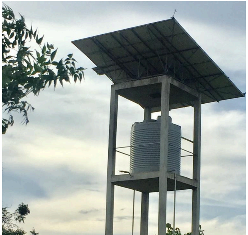
10-metre high solar-powered water tank in Namutumba, constructed to support irrigation agriculture.
