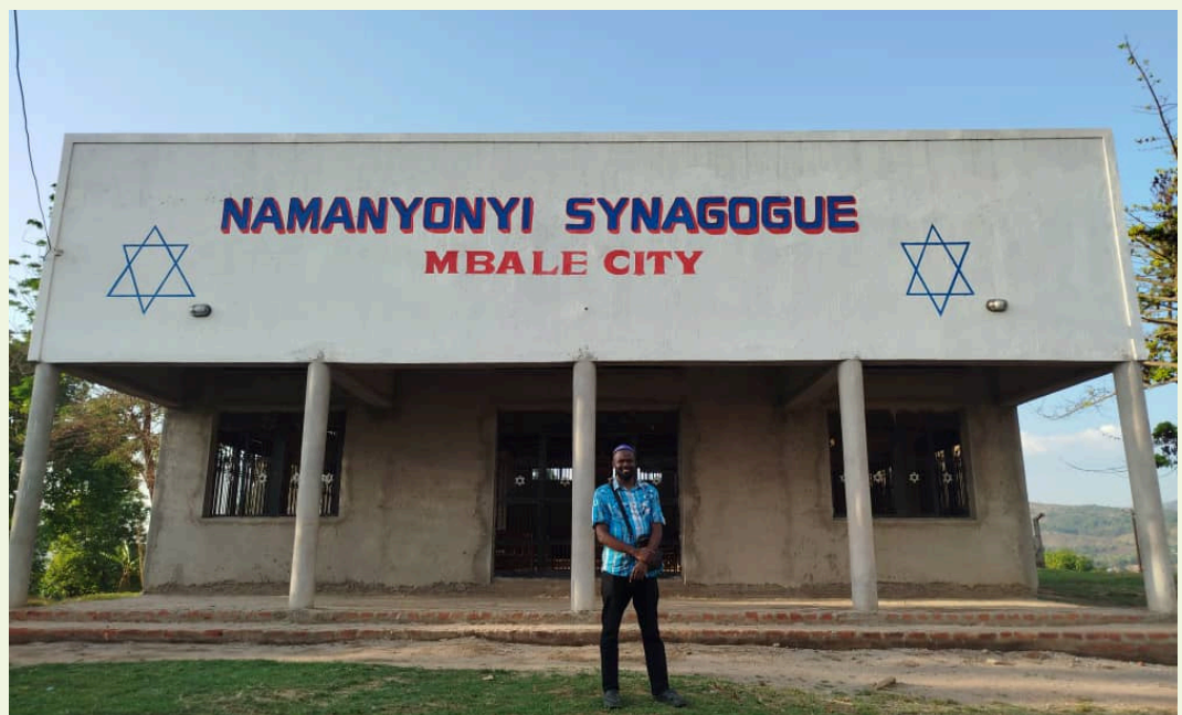
The newly constructed synagogue in Namanyoni — a modern structure designed to accommodate over 500 worshippers.
